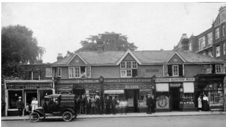
A row of Belgian shops in East Twickenham
