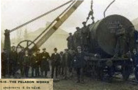
Top: Delivery of a boiler for the new factory at Twickenham Station.
